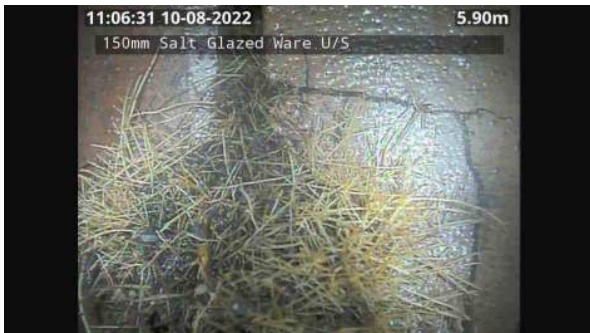
LS163731_21a34140-f995-4f12-b6d7-3720422e5b05_20220809_110746_244.jpg, 00:12:28, 5.90 Roots, at joint at 5 o'clock
