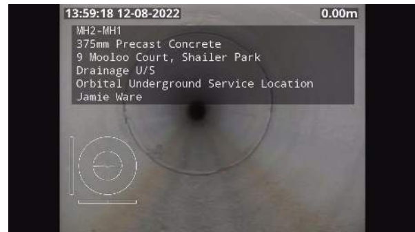
1_46e48fd8-da88-43c9-87d2-15a080f03879_20220811_140009_964.jpg, 00:00:22, 0.00 Water level, clear flow (the invert is visible), water level: 0%
