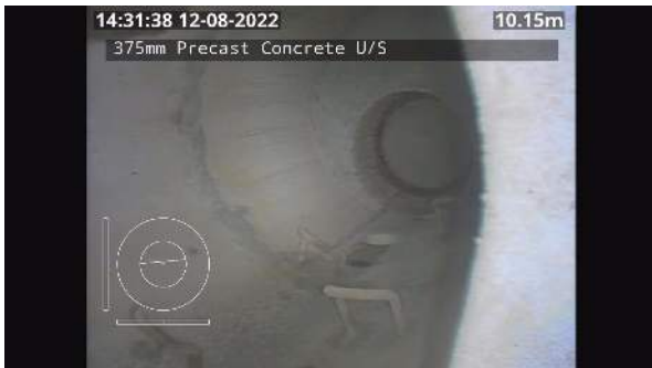
2_8575c63a-614f-48f5-8620-7e83d79b1442_20220811_143220_680.jpg, 00:05:54, 10.15 Finish node, maintenance hole, Nodename:, MH3
